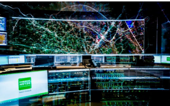
Monitoring the power grid in the network control room, photo: Energie Steiermark/Werner Krug
